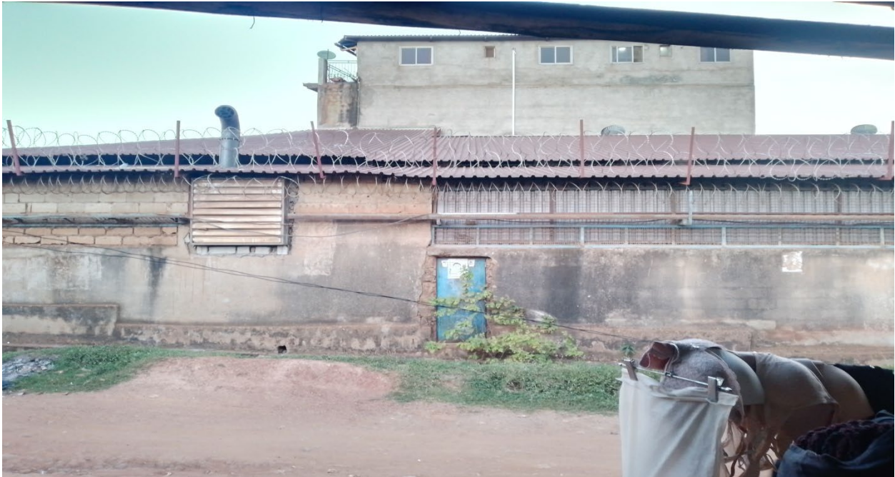
This is Biplous 'U' Ltd Factory. It reportedly emits itching smoke & loud noise in corner zone, Kawempe
