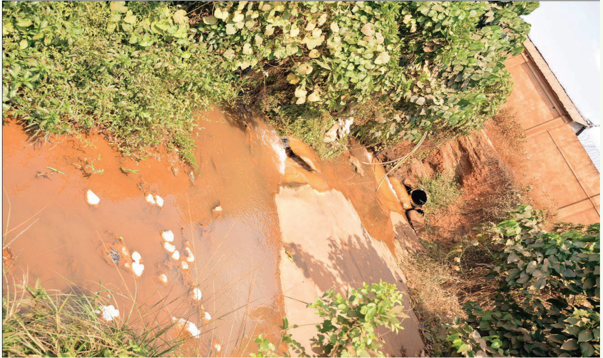
In the picture (above - centre right) is a pipe which local leaders said carries waste into Komamboga wetland from Tianyi Plastics Limited in Komamboga parish, Kawempe Division
